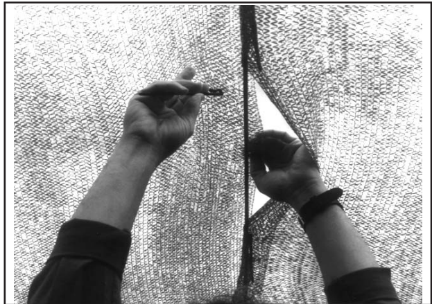
Fastening a net with a pin clip to the wire
